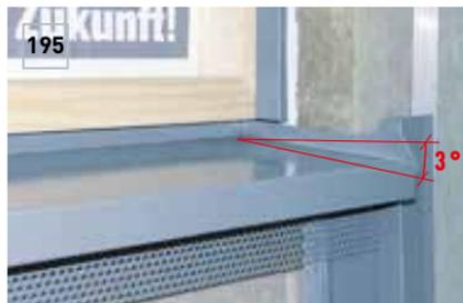
Push in the window ledge and mount the front fold in the window ledge flashing strip (Fig. 194 and 195).
