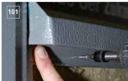
Allow a distance of at least 10 mm between the perforated plate and the window ledge (Fig. 99–101).
