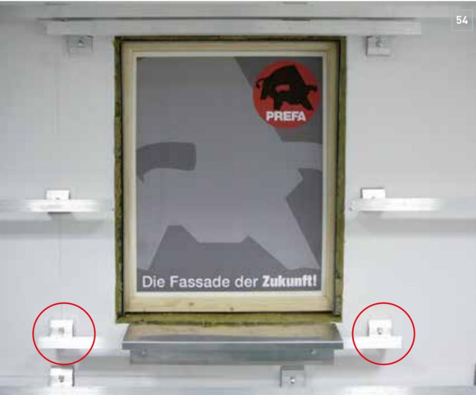
Fully installed window substructure with window ledge flashing strip.
