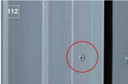
At the front, the siding is fastened between the siding and the window reveal by a riveted joint (Fig. 112).
