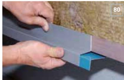
When attaching the drip, make sure that the installation is perfectly horizontal (Fig. 81).
