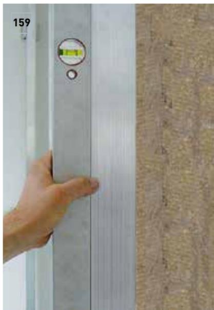
When fastening all the L-profiles, fasten one as a fixed point and all the others as sliding points (Fig. 160 and 161).
