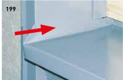
Then install the side reveal flashing on the window by inserting them into the interlocking profile. Fold down the window reveal at the bottom (Fig. 198 and 199).
