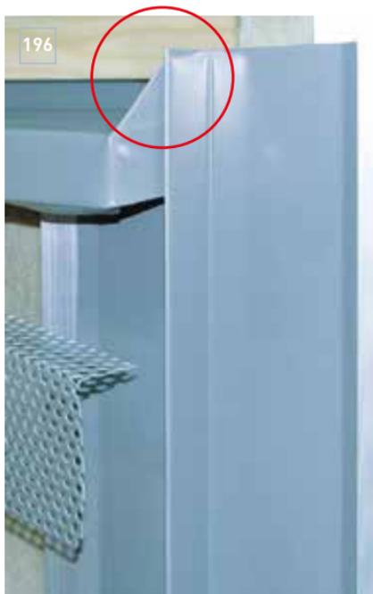
After mounting the window ledge, install the vertical joint connections under the window along the window reveals (Fig. 196 and 197).
