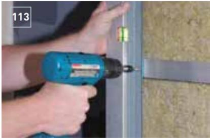
Mounting the reveal flashing on the right (Fig. 113).
