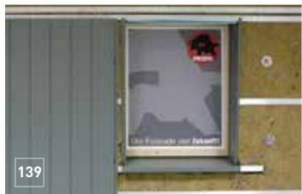
Now make the lateral and bottom window connections. In this design, the storey separation replaces the top window connection (Fig. 140).
