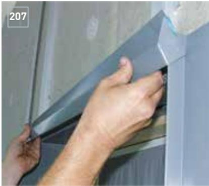
The prepared storey separation profile is mounted in the front part (perforated strips) of the reveal flashing, and fastened to the sub-structure (Fig. 207).
