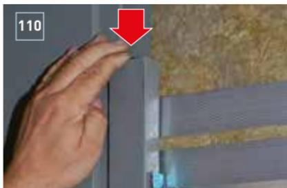
Fold the top end of the reveal flashing (Fig. 107).
