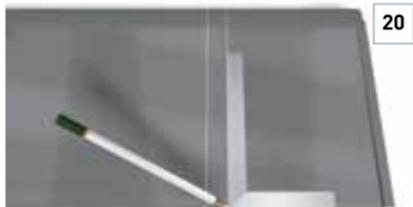
Due to the panel overlap, it may be necessary, to form a slightly tapered upstand.
