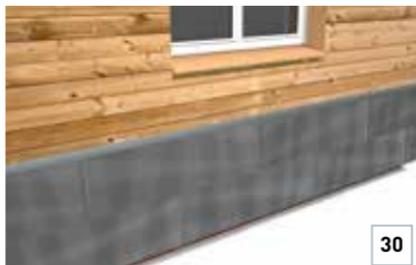
Make sure that the FX.12 panel is aligned horizontally.
