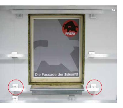
Fully installed window substructure with window ledge flashing strip.
