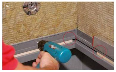
Aligning and fitting the perforated plate
