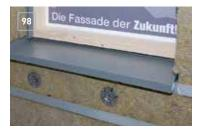
**Installing the window ledge** Push in the window ledge and mount the front fold in the window ledge flashing strip.
