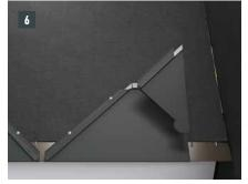
The sloping patent fold is to be notched at the top in the area of the raised edge corresponding to Image 6.
