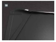
Open the upper panel fold of the PREFA roof covering and raise the roof covering 30 mm up to the 90° mark (Image 5A + 5B).
