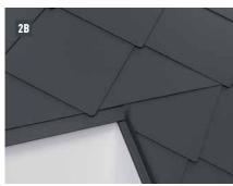
The following row of rhomboid roof tiles can then be installed over the entire width (Image 2A + 2B).
