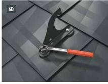
¬ Mounting of the mountain snow guard support with both hexagon head screws (M12) to the foot parts (SW 19; torque: 35 Nm) for roof tiles (Image 6A), roof shingles (Image 6B), rhomboid roof tiles (Image 6C), R.16 and FX.12 (Image 6D).
