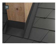
Prepare the surroundings (back and side part) and fix these to the side parts of the substructure with return clips.
