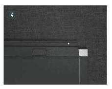
Notch the upper patent fold in the area of the raised edge so that a hook fold remains and bend the R.16 roof tile or the FX.12 roof panel upwards 30 mm at a right angle to the roof surface (Image 3 + 4).
