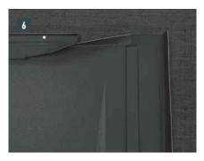
When edging backpart, the upper hook-on seam of the R.16 roof tiles or FX.12 roof panels to be covered is cut at approx. 200 mm and notched. The hook-on seam is bent backwards and the side overhang is bent up 90° (Image 5 + 6). The back part of the surroundings to be installed.
