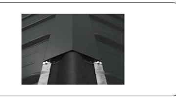
Figure 73 - Ridgedetail with simple ridge cap
