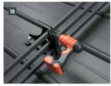
Fasten each insert profile once in thecentre of the profile length with the supplied  $5.5 \times 25$  mm TX25 self-tapping screws (1 pc. per insert profile) to prevent lateral shifting of the bars and to ensure profile expansion to the left (Image 9 + 10).
