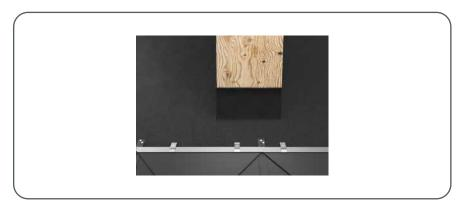
Figure 105 • Chimney edging - 29×29 and 44×44 rhomboid roof tile - front part
