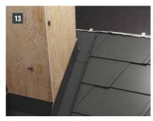
Place the vertical folds of the side parts in the upper area and trim the back part and the side parts with an allowance of 30 mm. Make the cover - now the covering of the roof surface above the surroundings can be continued.
