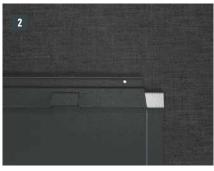
Notch the upper patent fold in the area of the raised edge so that a hook fold remains and bend the R.16 roof tile or the FX.12 roof panel upwards 30 mm at a right angle to the roof surface.
