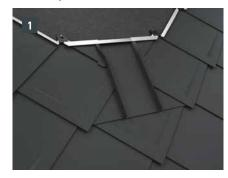
For the installation of an base plate, start and end plates must be laid with  $29 \times 29$  or  $44 \times 44$  rhomboid roof plates.
