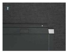
Notch the upper patent fold in the area of the raised edge so that a hook fold remains and bend the R.16 roof tile or the FX.12 roof panel upwards 30 mm at a right angle to the roof surface (Image 1 + 2).
