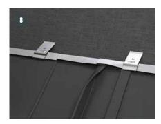
¬ Trim the neck part of the roof hatch along the course of the PREFA roof covering, fold over and fasten with clips (Image 8).
