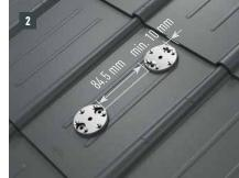
¬ Mark the centre of the rafter. The upper foot part (outer edge) should have a distance of at least 10 mm to the overlying fold. Observe distance (measured on the inside) of 84.5 mm between the two foot parts. For attachment to the rafter, the drill holes (∅ 8.5 mm) must lie on the axis of the snow rake hook (= course of the rafter) - Fixing screws in one axis with the rafter. Remove rear protective film on the foot parts, position and stick on (Image 1 + 2).
