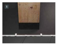
Pull up roof shingle and DS.19 shingle until the last row of PREFA roof covering can be covered under the chimney.
