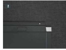
Notch the upper patent fold in the area of the raised edge so that a hook fold remains and bend the R.16 roof tile or the FX.12 roof panel upwards 30 mm at a right angle to the roof surface.
