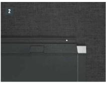
Notch the upper patent fold in the area of the raised edge so that a hook fold remains and bend the R.16 roof tile or the FX.12 roof panel upwards 30 mm at a right angle to the roof surface (Image 1 + 2).
